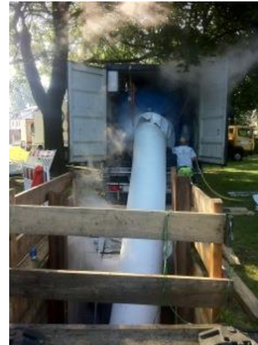
Liner inversion and steam curing
